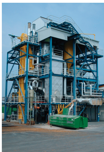
Güssing, Austria, wood gas project, 1x JMS 620
