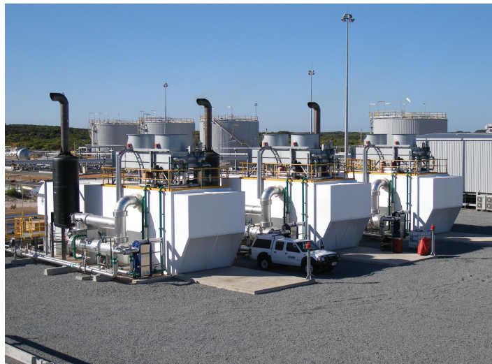
Cliff Head, flare gas project, Dongara, Australia, 3 x JMS612
