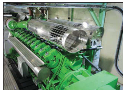
Fig. 5: Jenbacher engine installed on site. (photo credit SACC).
